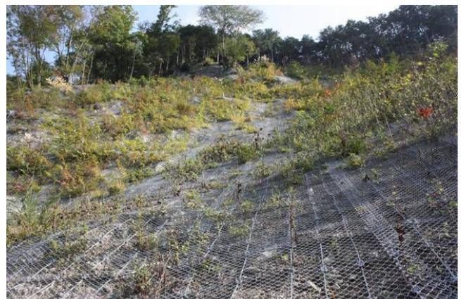
図4.17 覆式落石防護網
